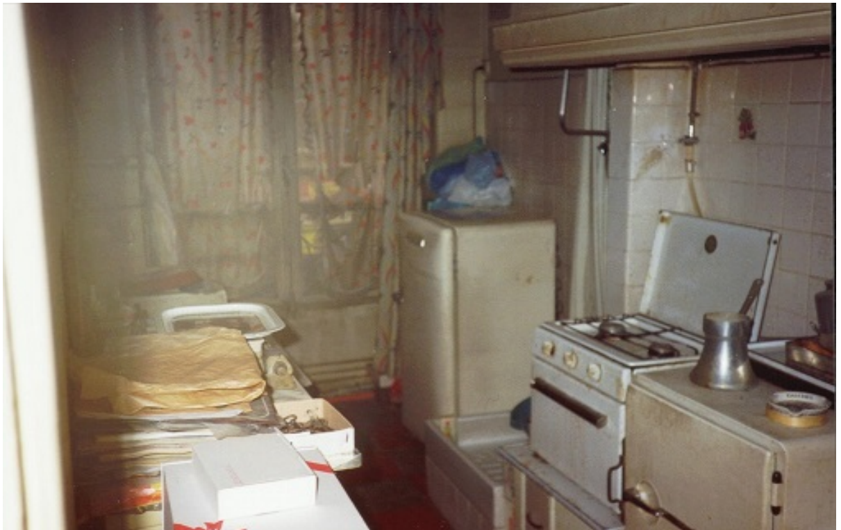
27 rue Oberkampf BEFORE remodeling - kitchen
